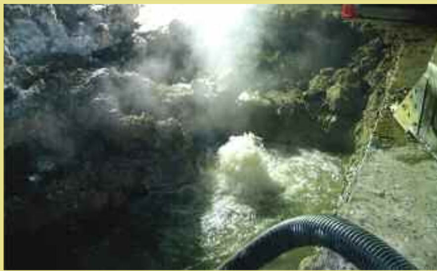
MMSD 36" Forcemain Repair — Monona, WI
