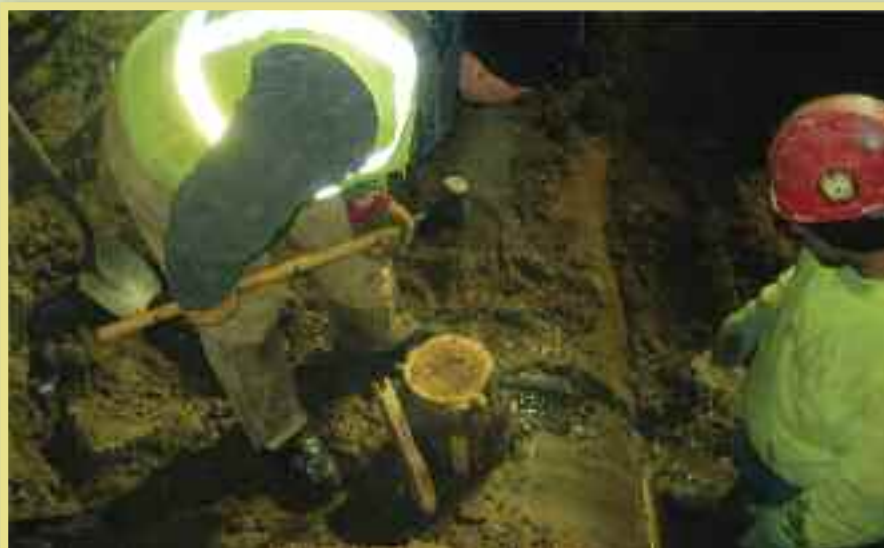
MMSD 36" Forcemain Repair — Monona, WI
